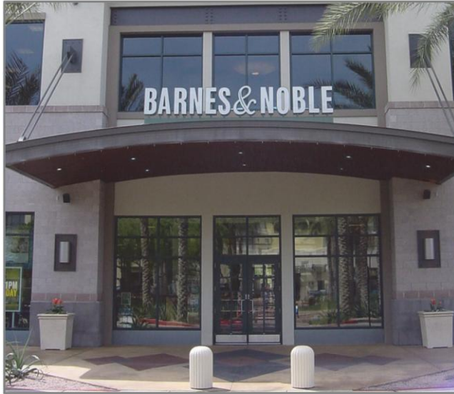
Photo: Canopy Sign
